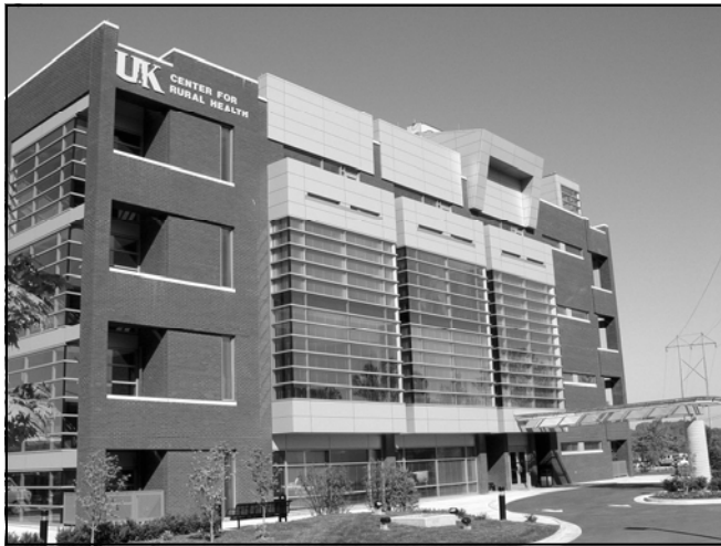
The UK Center for Rural Health Bailey-Stumbo building houses programs for Hazard Community and Technical College. Nursing, Radiography, and Physical Therapist Assistant classes and faculty offices are located in this facility, located on Morton Blvd. in Hazard near Hazard ARH Regional Medical Center.
